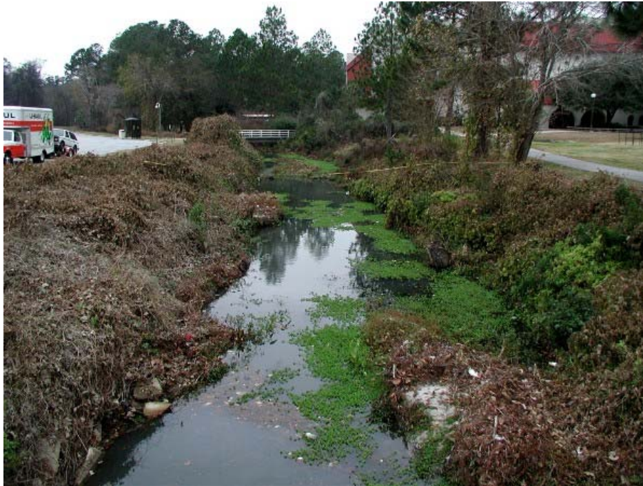
Figure A.21. Reach 4 at Cross Section B Facing Downstream, January, 2004.
