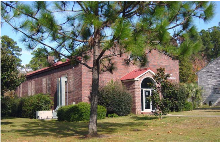
Warehouse NC1 North Campus
